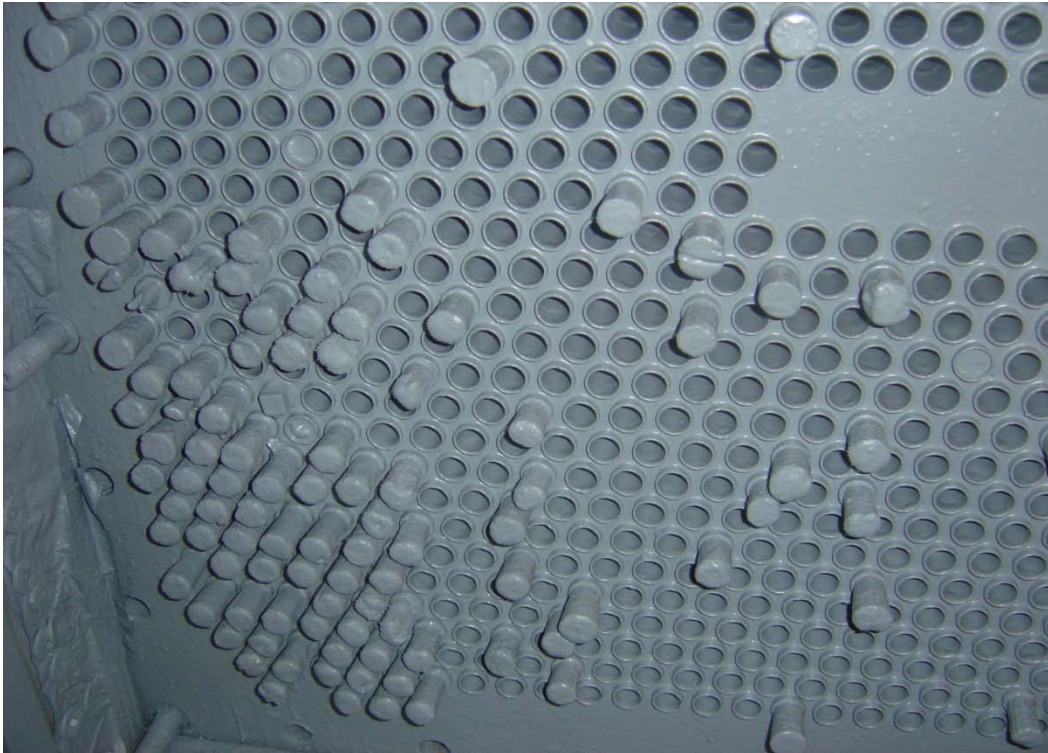
Condenser tube sheet and tubes after application of coating (tube lining)
