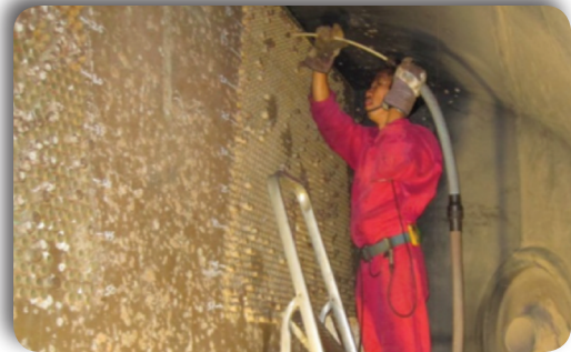
Condenser tube ID cleaning and ECT inspection
