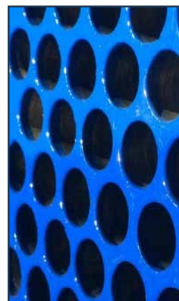
Tubesheet restoration complete using Curran International's polymeric epoxy cladding system.
