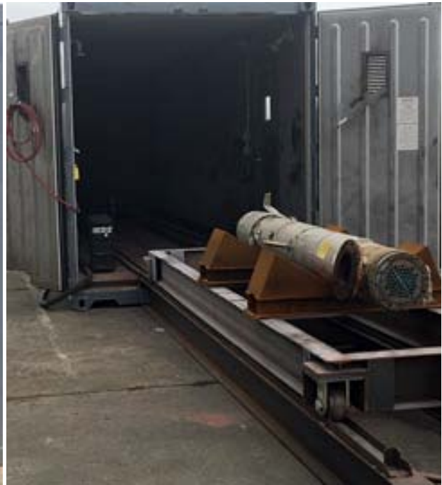
A small exchanger is on V-block and ready to roll into the blast module. Two bundles can be loaded at the same time. When blasting the end doors are closed, sealing all blast-waste inside.
