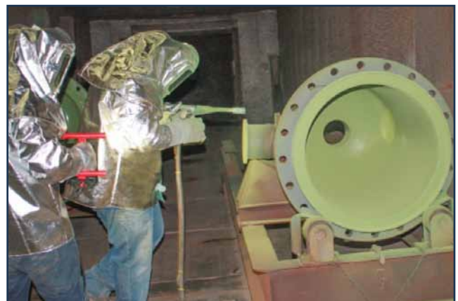
Curran techs applying PTFE coating using "hot flock" method
