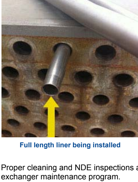
Full length liner being installed
