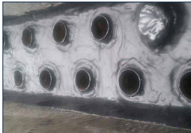
Tube Plate After Coating
