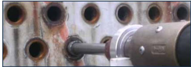
Curran specialized nozzles "bridge" and capture waste-grit and tube debris tube-end to tube-end.
