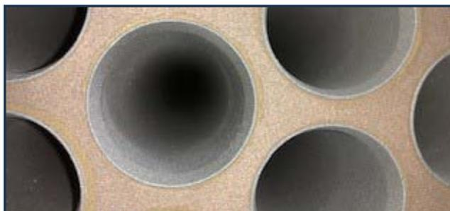
Curran grit blast surface preparation of tube ID and tubesheet yielded clean surface for coating.
