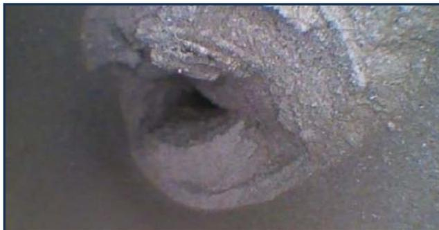
Salt water sediment and deposits severely fouled many of the condenser tubes requiring hydro lancing to clear.
