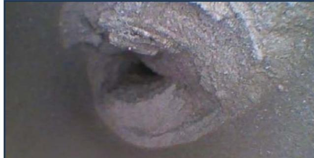
Salt water sediment and deposits severely fouled many of the condenser tubes requiring hydro lancing to clear.
