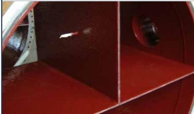
A 46”-diameter cooling water channel. Curran coated for return to service. Stainless steel anode lugs were masked where already installed. Curran clients find extended life of anodes when combined with coating.
