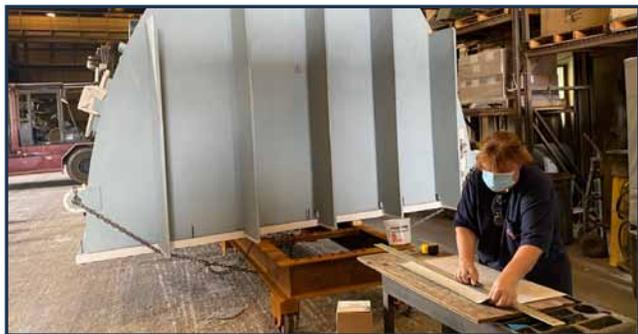
Power plant waterbox internal coating; Curran technician preparing blast mask to protect gasket sealing surfaces prior to grit blast surface prep and application of Carboline epoxy.
