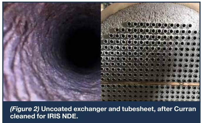
(Figure 2) Uncoated exchanger and tubesheet, after Curran cleaned for IRIS NDE.
