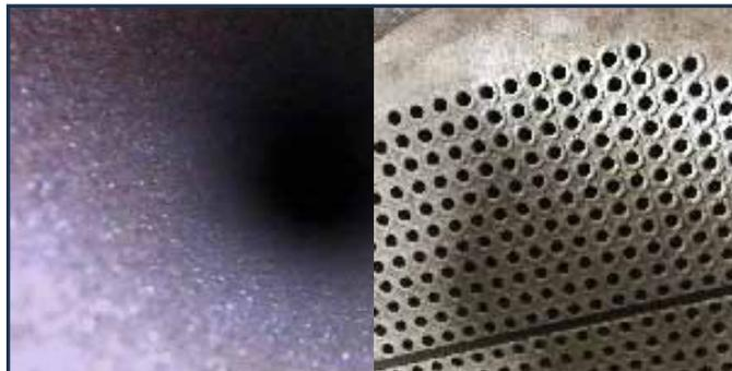
(Figure 1) Formerly coated exchanger and tubesheet, after Curran cleaning and coating removal for IRIS NDE.
